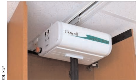
Figure K-8: Recessed Track
