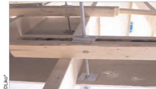
Figure K-11: Threaded Rod Mount
